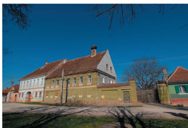
Habitations complexes à côté de la Place (rue Morii) Large residences in the Market Place neighbourhood (Morii street)
