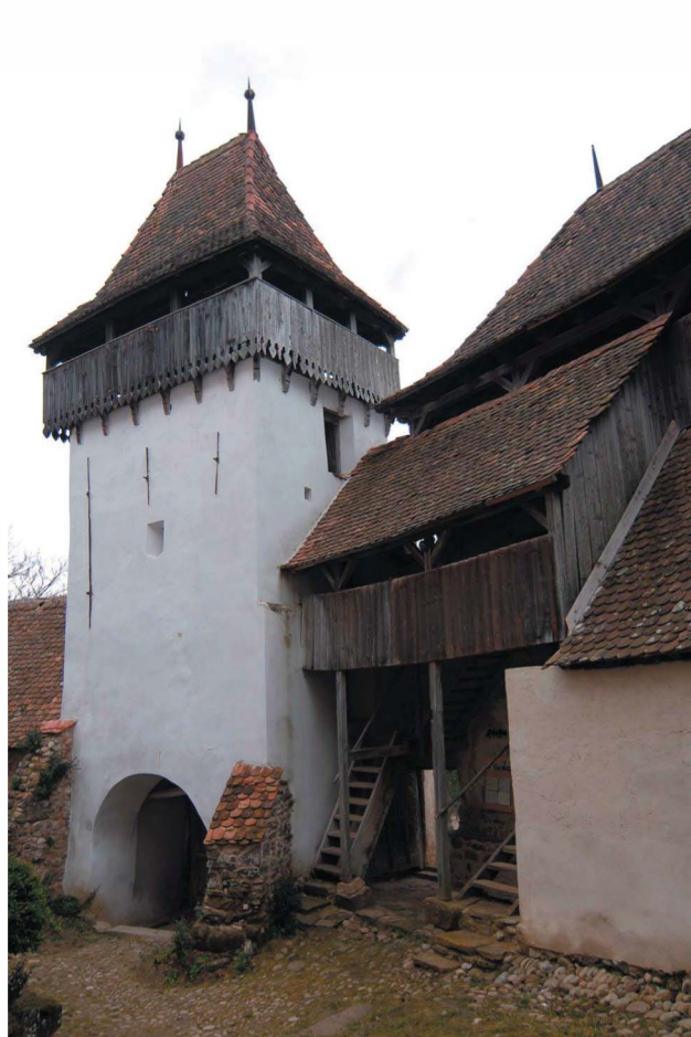
La tour porte et le bastion sud The gate tower and the south bastion
